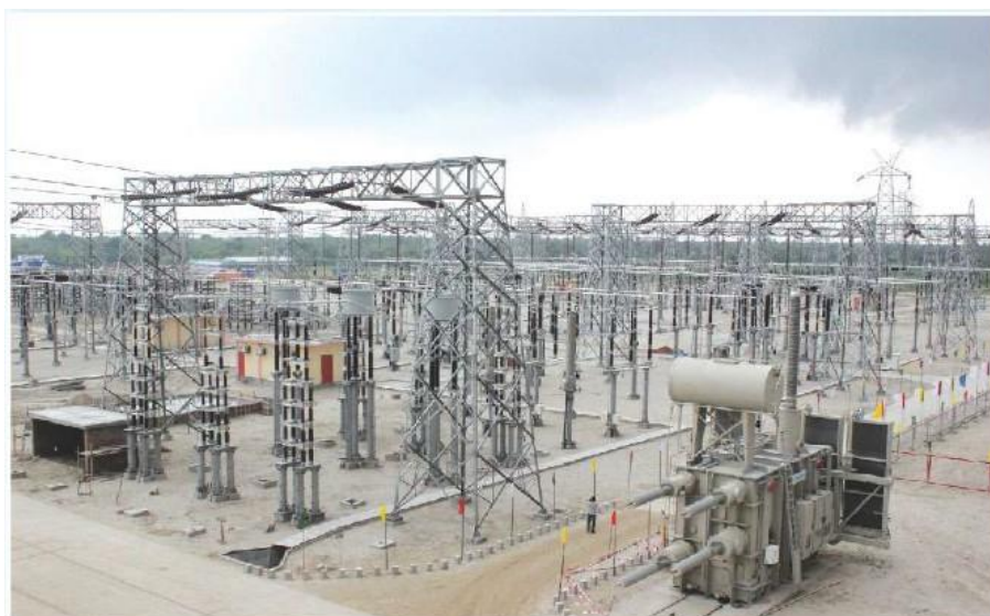
Figure 20: Bangladesh India Power Transmission Plant, Bheramara (Kustia)
