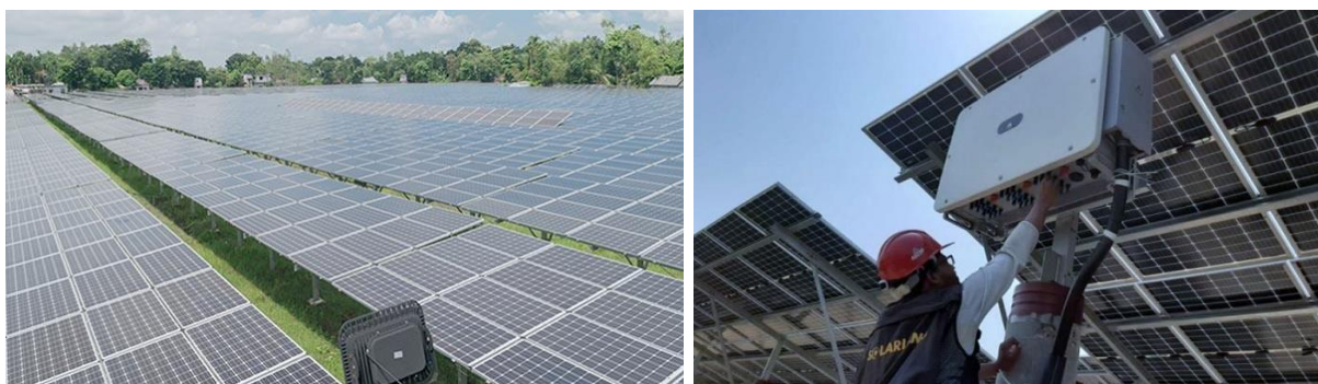
Figure 24: Bangladesh's Largest (73 MW) Solar Power Plant, Mymensingh
